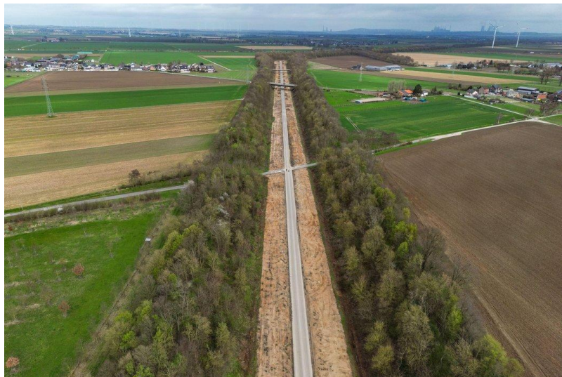
Route of the Rhine water transport pipeline to flood the Hambach and Garzweiler mines to create new lakes (credit: Oliver Berg/dpa/Alamy Live News)
